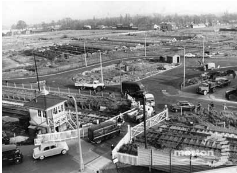
Eastfields level crossing 1961
