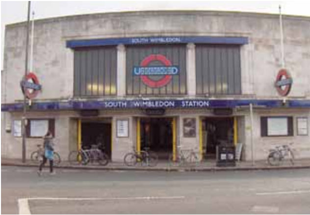
South Wimbledon underground station
