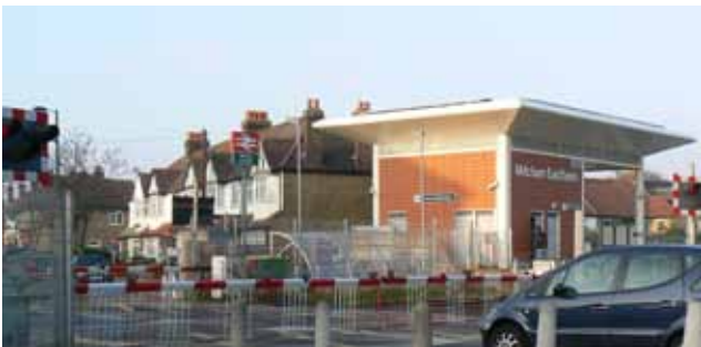
Level crossing at Mitcham Eastfields station
