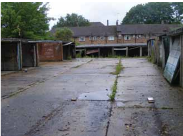
Later addition: Ravensbury garages
