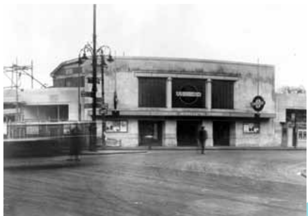
South Wimbledon station 1926
